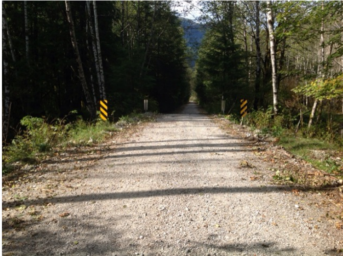
Approach from Left Bank when facing downstream
